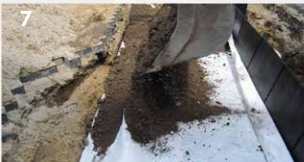
7 Apply geotextile and backfill with mixed aggregate
