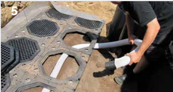
5 Install the aeration and irrigation system
