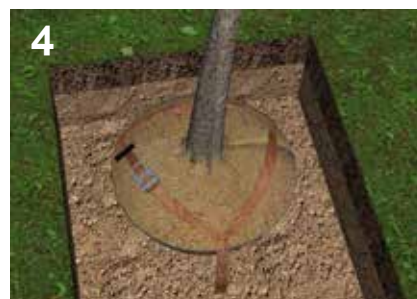
4 Tighten the strap by winding the ratchet. Repeat after 2 days, after tightening unhook the ratchet tensioner.
