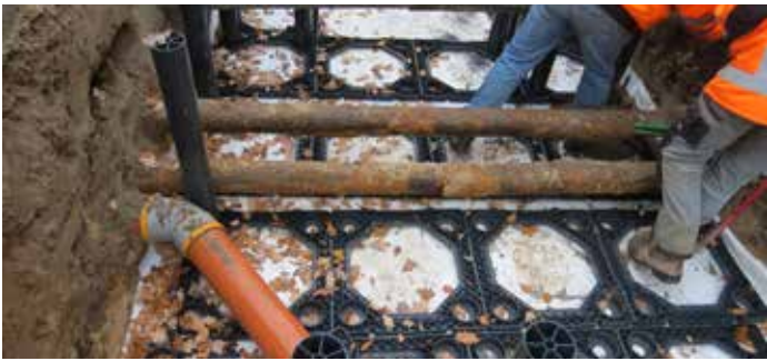
TreeParker® is easy to install, even around cables and pipes. For more information, see manual 'cables & pipes TreeParker® in the city'
