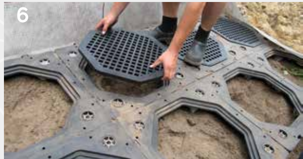
6 Closing the system with decks
