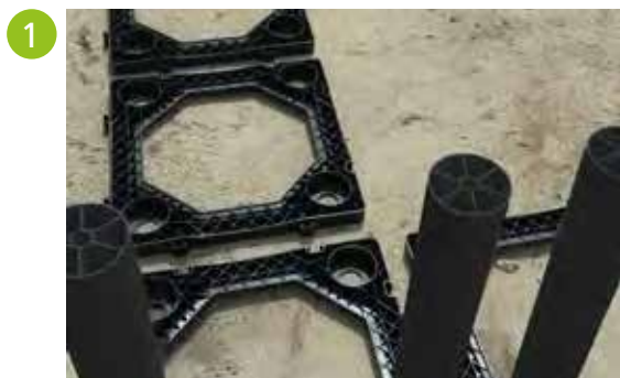
1 Place the frames around the treepit opening
