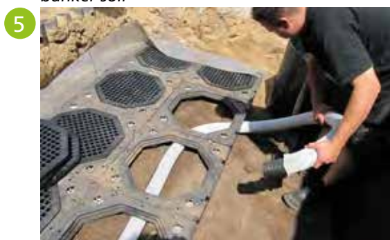
5 Install (deep-) aeration / irrigation systems
