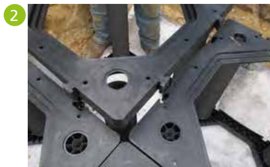
2 Attach the posts and top frames
