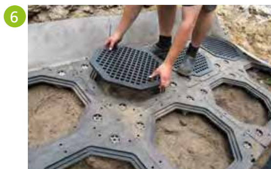
6 Closing the system with decks
