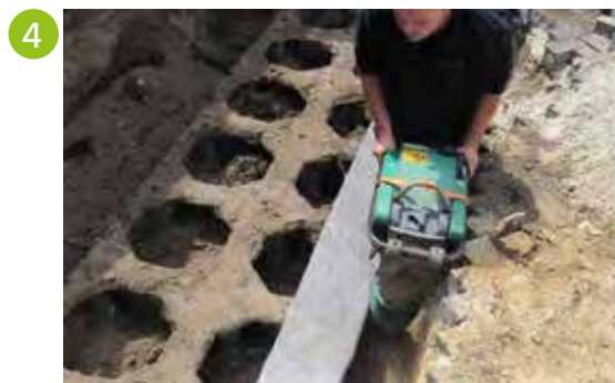
4 Fill / compact around the system
