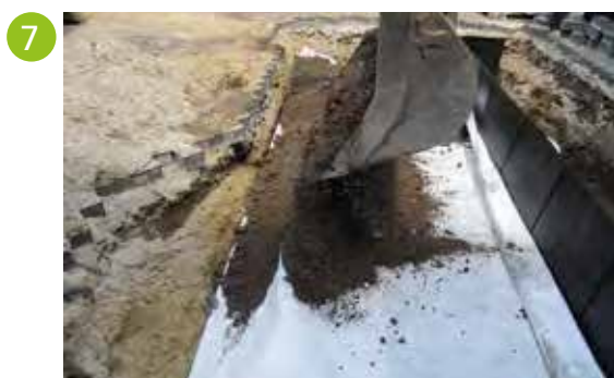
7 Apply geotextile and fill with mixed granulate
