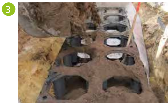
3 Fill the system with bioretention soil / tree bunker soil
