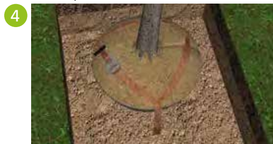
Tighten the strap by winding the ratchet. Repeat after 2 days, after tightening unhook the ratchet tensioner
