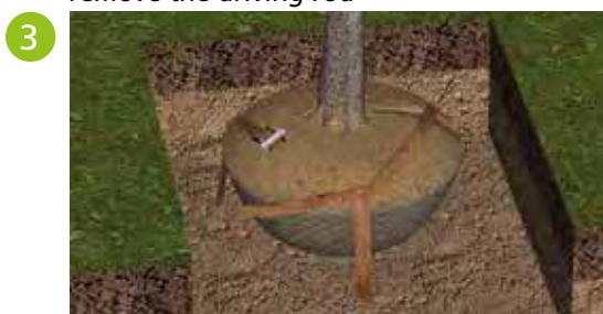
Push the tensioning strap through the 3 loops
